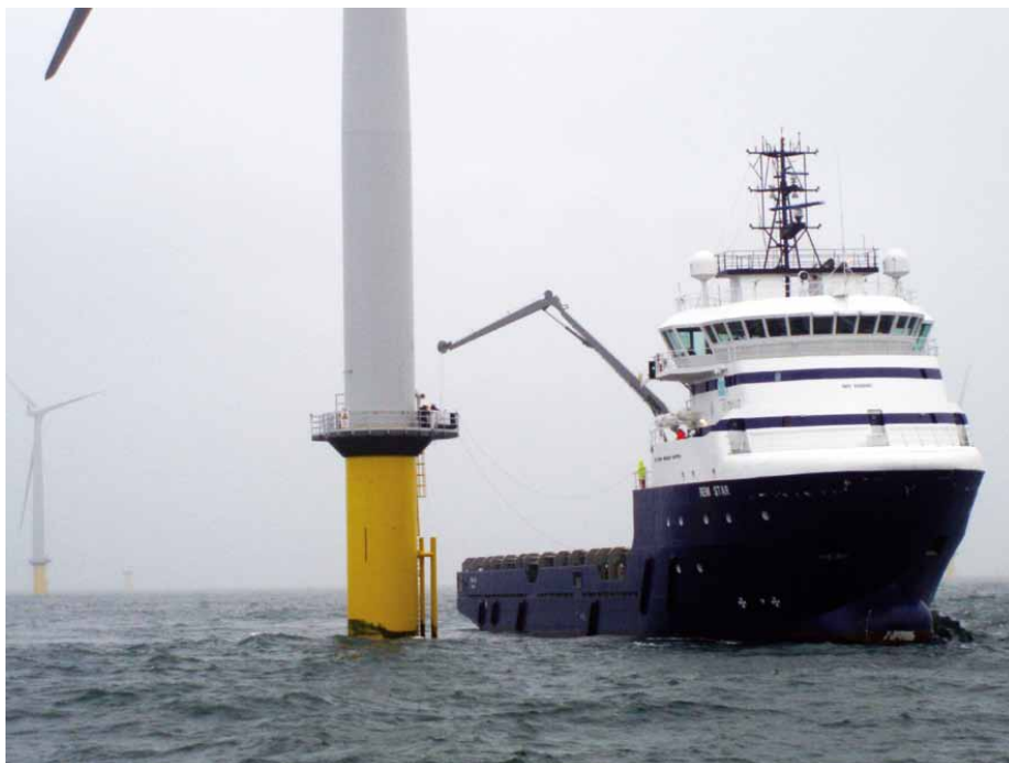
A2Sea is involved in the installation of approximately 60% of the world's windmills at sea.
